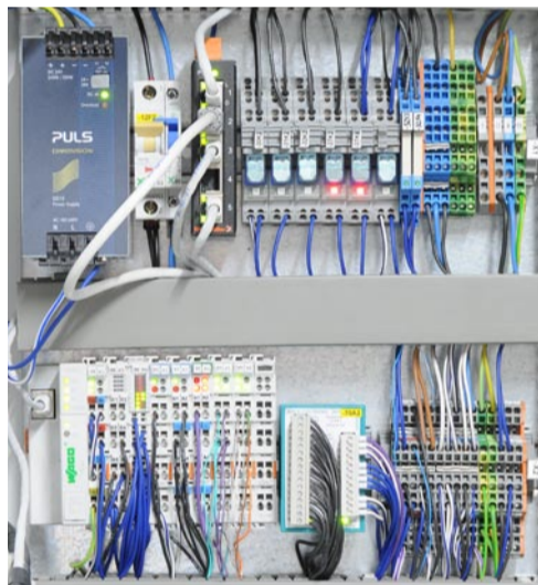
Frei programmierbarer Ethernet-Controller.
